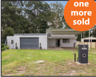
71 Waratah Crescent, Sanctuary Point
